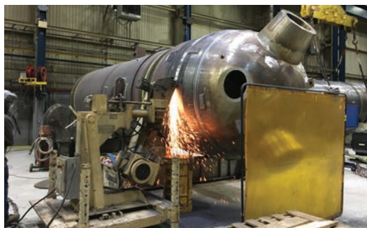
Right: BWXT Canada Inc. is manufacturing 32 steam generators at its Cambridge facility for Bruce Power's major component replacement
