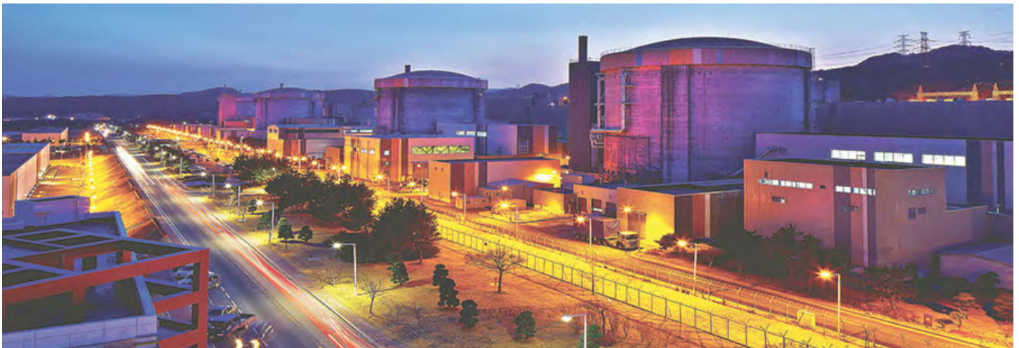
COG is currently supporting KHNP, Korea in the development of a decommissioning schedule for Unit 1 at its Wolsong plant (pictured). Image: KHNP
