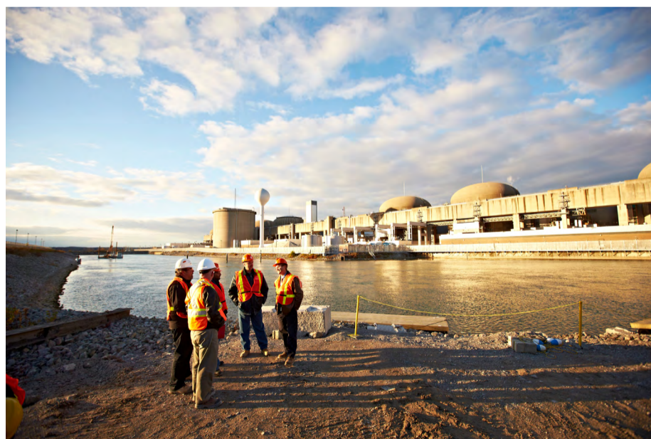
As more CANDU reactors, like Pickering Nuclear, above, approach end of operation, COG and its members are increasingly looking to develop innovative approaches to decommissioning and waste. COG's enhanced agreement with the IAEA will further collaborative efforts in these and other areas. Image: OPG
