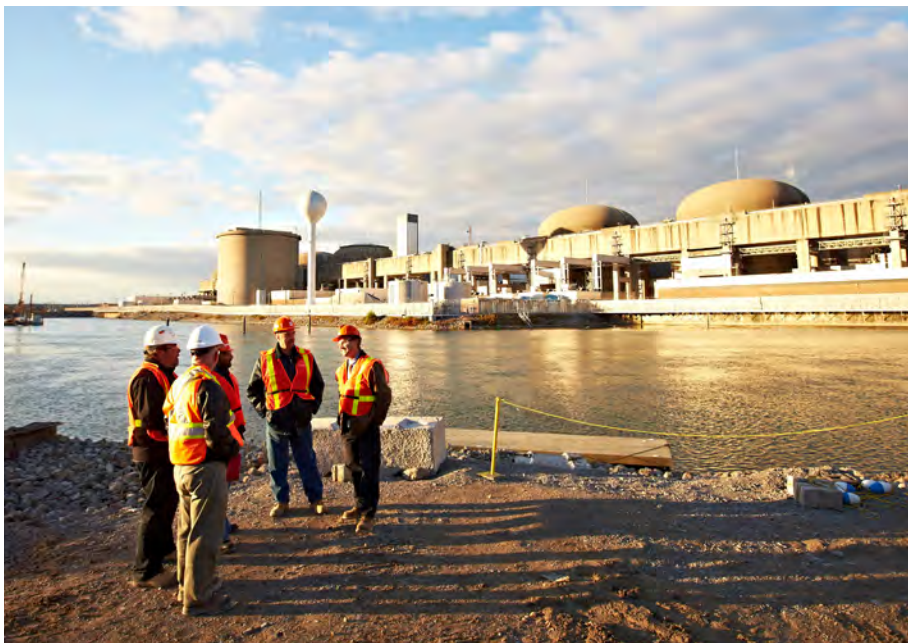
As more CANDU reactors, like Pickering Nuclear, above, approach end of operation, COG and its members are increasingly looking to develop innovative approaches to decommissioning and waste. COG’s enhanced agreement with the IAEA will further collaborative efforts in these and other areas. Image: OPG
